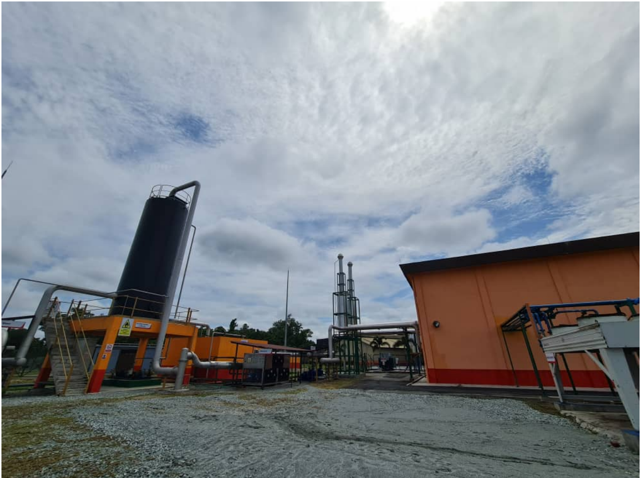
FGV's Triang biogas power plant building
