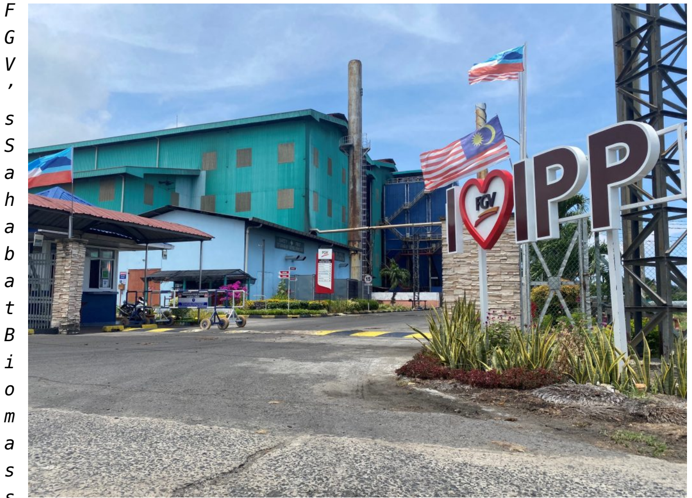
Cogeneration Plant in Lahad Datu, Sabah
